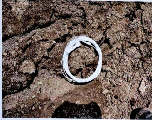
Gambar 23. Surface Delay
