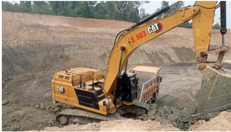
Gambar 10 Kondisi Aktual Fleet 2 Overburden
